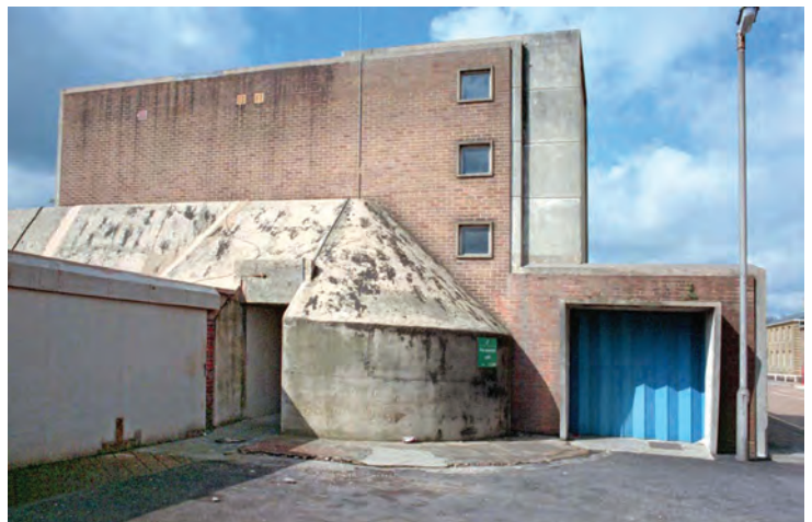
The new dock telephone exchange was built on top of the bunker in 1958. The building on the left is also a later addition. The entrance in the corner of the bunker is into the Southampton Docks control room.
